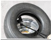
Pull the handle to an upright position to start the bottom bead over the edge of the rim.
